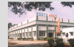
Roots Multiclean Ltd., Coimbatore, India
